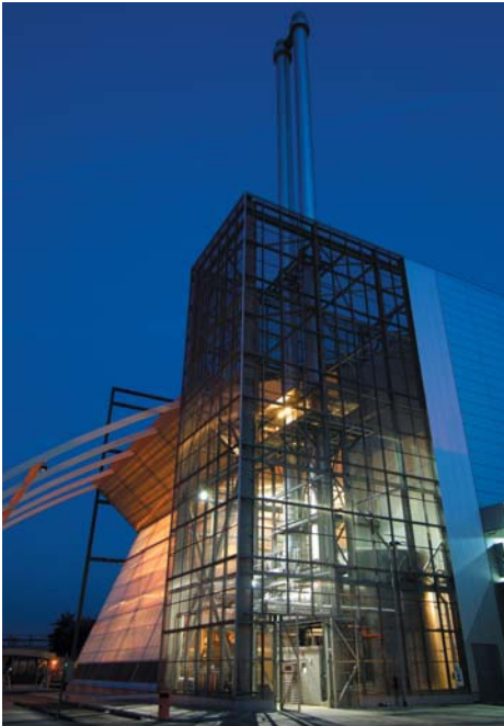
Portsmouth ERF, Portsmouth, United Kingdom 165,000 Tonnes Per Year
