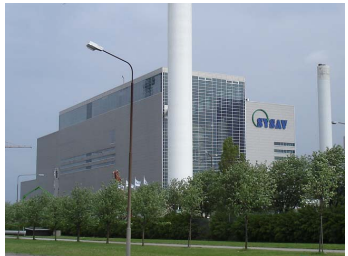
SYSAV Waste to Energy Plant, Malmö, Sweden 600,000 Tonnes Per Year
