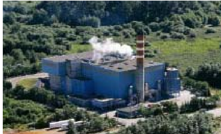
Greater Vancouver Regional District's Waste to Energy Facility, Burnaby, British Columbia 250,000 Tonnes Per Year
