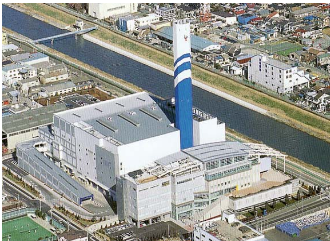
Asahi Clean Centre, Kawaguchi City, Japan 135,000 Tonnes Per Year
